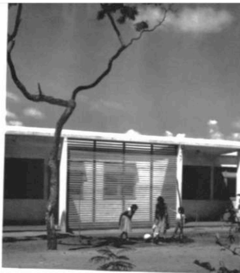
107. Row Houses, Brasília, 1958. A dwelling unit
