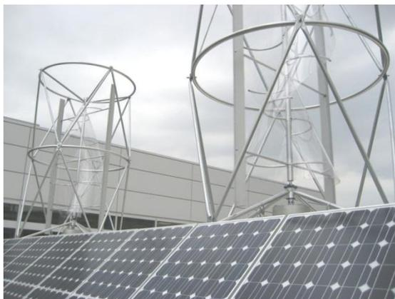
**Figura 63 - Aerogerador Aerotecture instalado no topo do International Brotherhood of Electrical Workers (IBEW). Fonte: (AEROTECHTURE INTERNACIONAL INC., 2010).**
