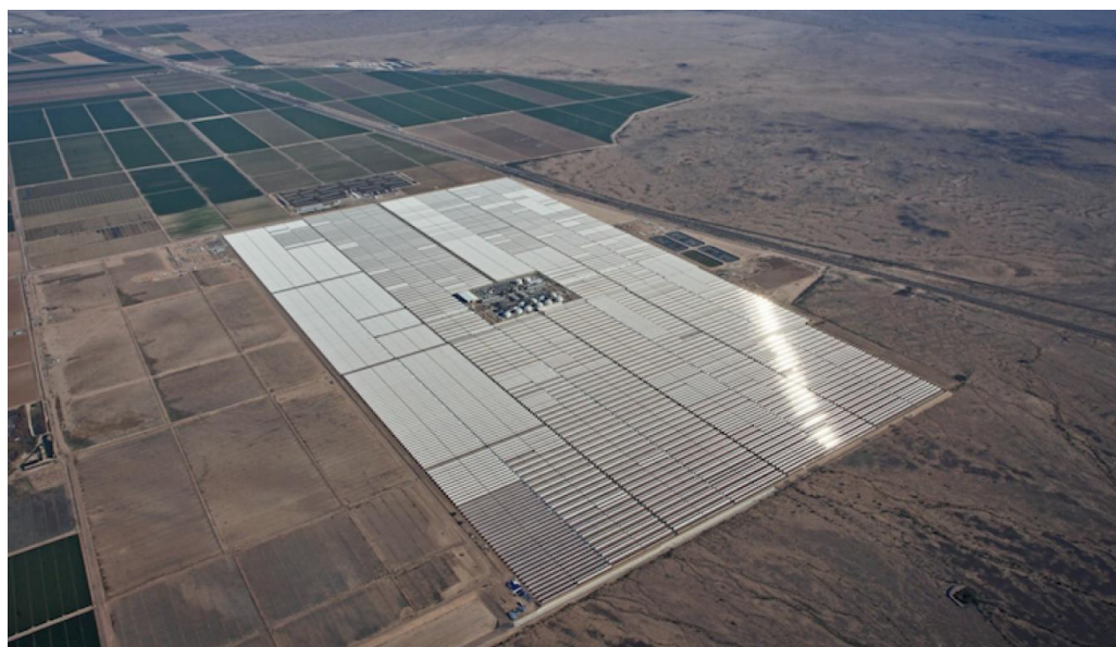
Figura 6: Solana Generating Station.
