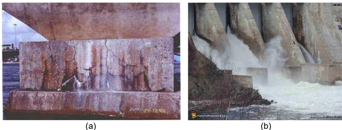
Figure 3.2 – Structures affected by ASR in which the aggregates evaluated in this study were used. (a) Paulo Guerra bridge, Recife, Brazil (Mylonite). (b) Mactaquac dam, New Brunswick, Canada (Springhill).
